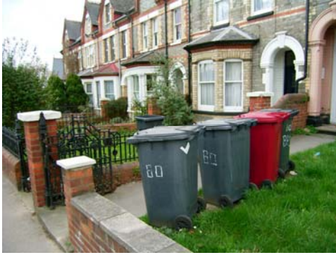
This example of existing development highlights problems arising from development of flats..
