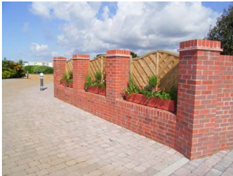
Here thought has been given to providing a well screened, accessible store for recycling and waste bins.
