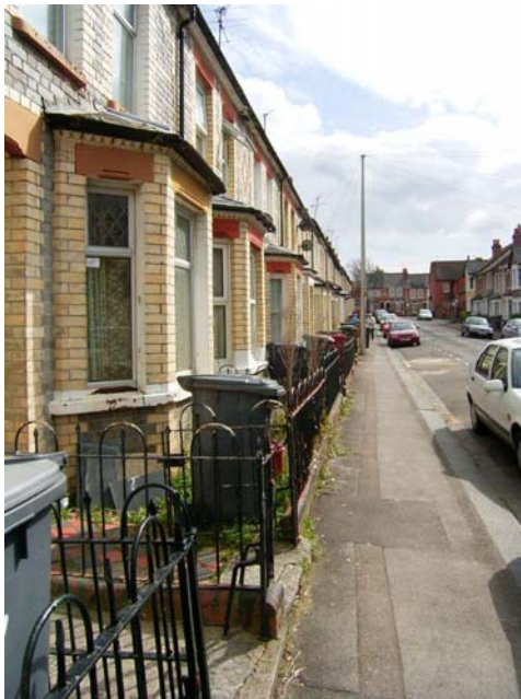
Shallow frontages in a traditional 19th Century terrace leaves limited scope for successful integration of bins .....
