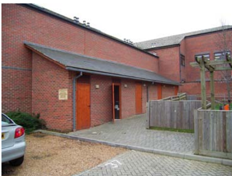
A series of enclosed binstores for a multiple flat development have been built against an otherwise blank wall. The enclosing structure picks up reference particularly in terms of materials from the main development.
